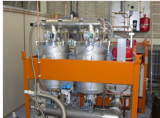
Figure 1 The SOCOOL Tri - generation system under construction
