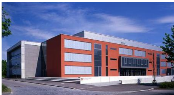
Main building (S-W elevation), as seen from Leipziger Strasse [(C) Elwert & Stottele]
