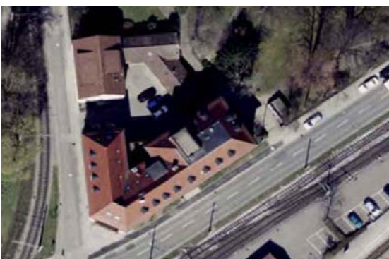
The nursery before retrofitting
