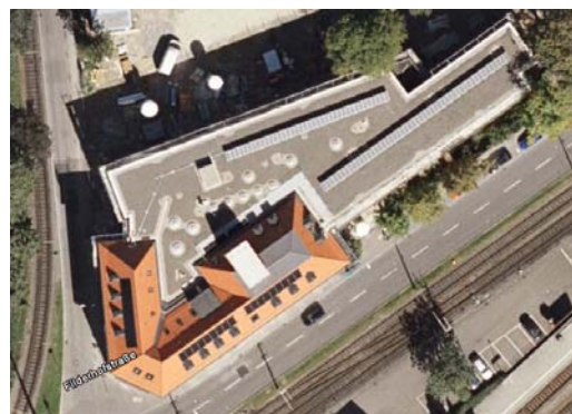
The nursery after retrofitting
