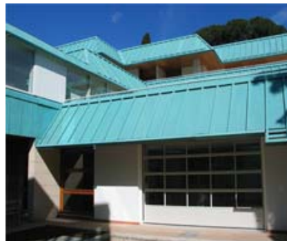
Sun shading systems used for patient rooms and the greenhouse
