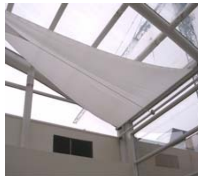
Sun shading systems used for patient rooms and the greenhouse
