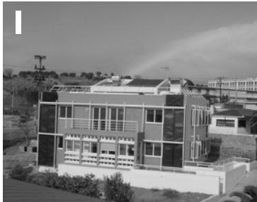
Picture 1: Solar air collectors, 25m 2 , placed south façade on the bioclimatic building of CRES coupled to a 16.7 kW air sourced heat pump.
