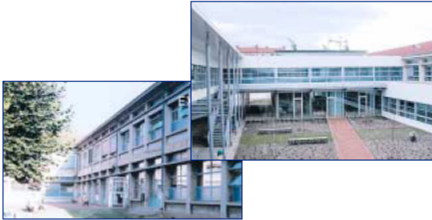
Left: Patio Before Refurbishment / Right: Patio After Refurbishment
