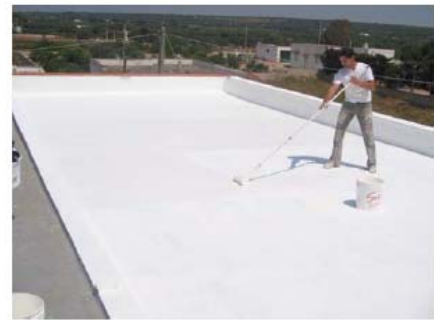
White paint on a flat roof
